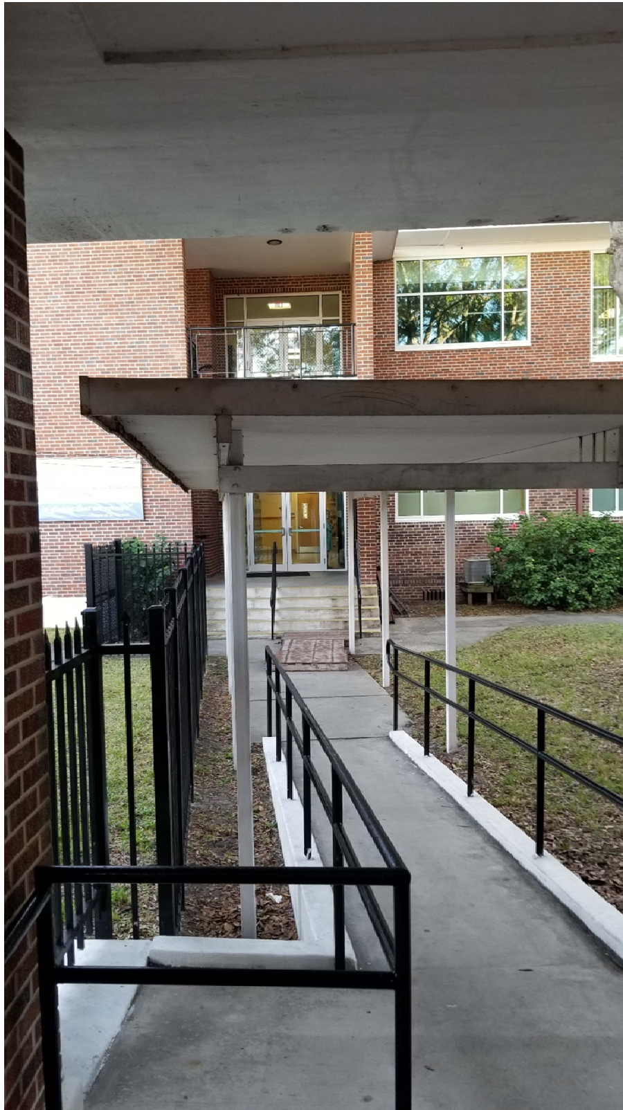
6. Breeze Way Facing East
