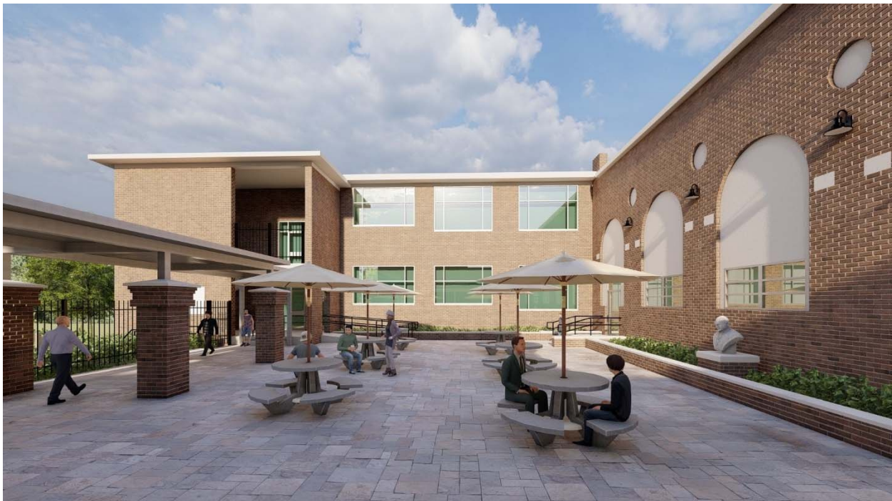
4. Courtyard Facing East
