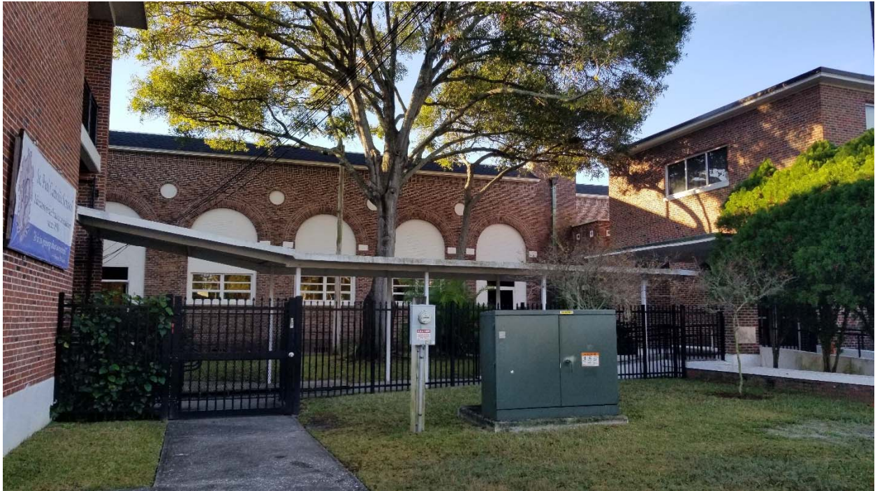
1. North Façade Eastern Entrance
